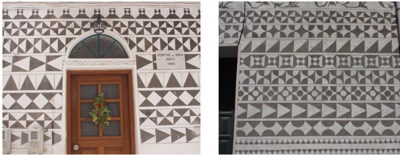
Figure 2: Photos from houses in Pyrgi, Chios, Greece.
